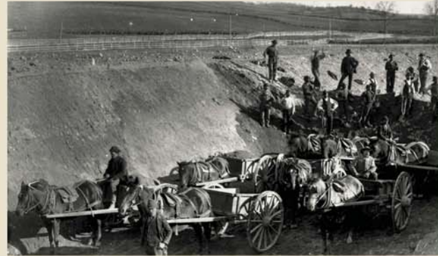
Late nineteenth-century railroad line construction in Dutchess County
