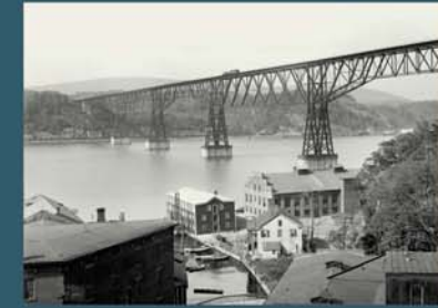
The Poughkeepsie Bridge in the early 1900s
