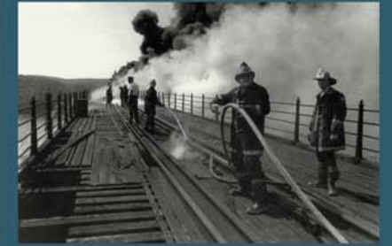
Firefighters attempt to put out the fire on the bridge
