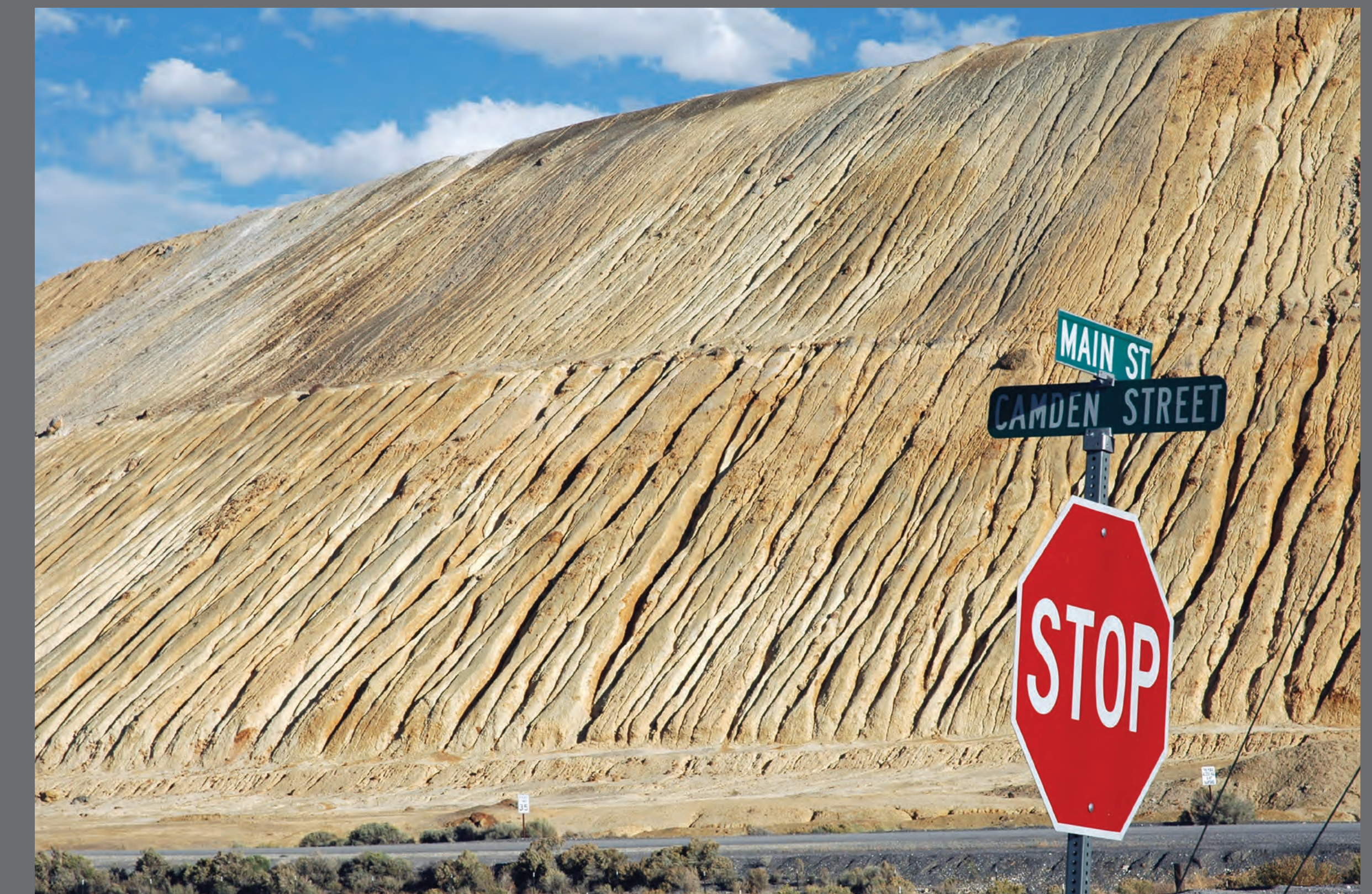
KEYSTONE MEMORIES Kennecott Copper stopped dumping waste rock at Keystone Dump in 1958. Further expansion was blocked by existing roads and Nevada Northern Railway lines running along the sides of the dump, which then contained 94 million tons of material covering 190 acres. Over the next sixty years of exposure to the elements, Keystone Dump waste rock softened and its slopes eroded, taking on a corrugated texture that became familiar to travelers on U.S. Route 50 and Ruth residents, miners, and visitors. The historic Keystone Dump symbolized over 100 years of human effort and changing landscape. KGHM’s changes to the Keystone Dump landscape are part of another chapter in Ruth’s rich mining history. Source: Milestone Heritage Consulting / Matt Kierstead
