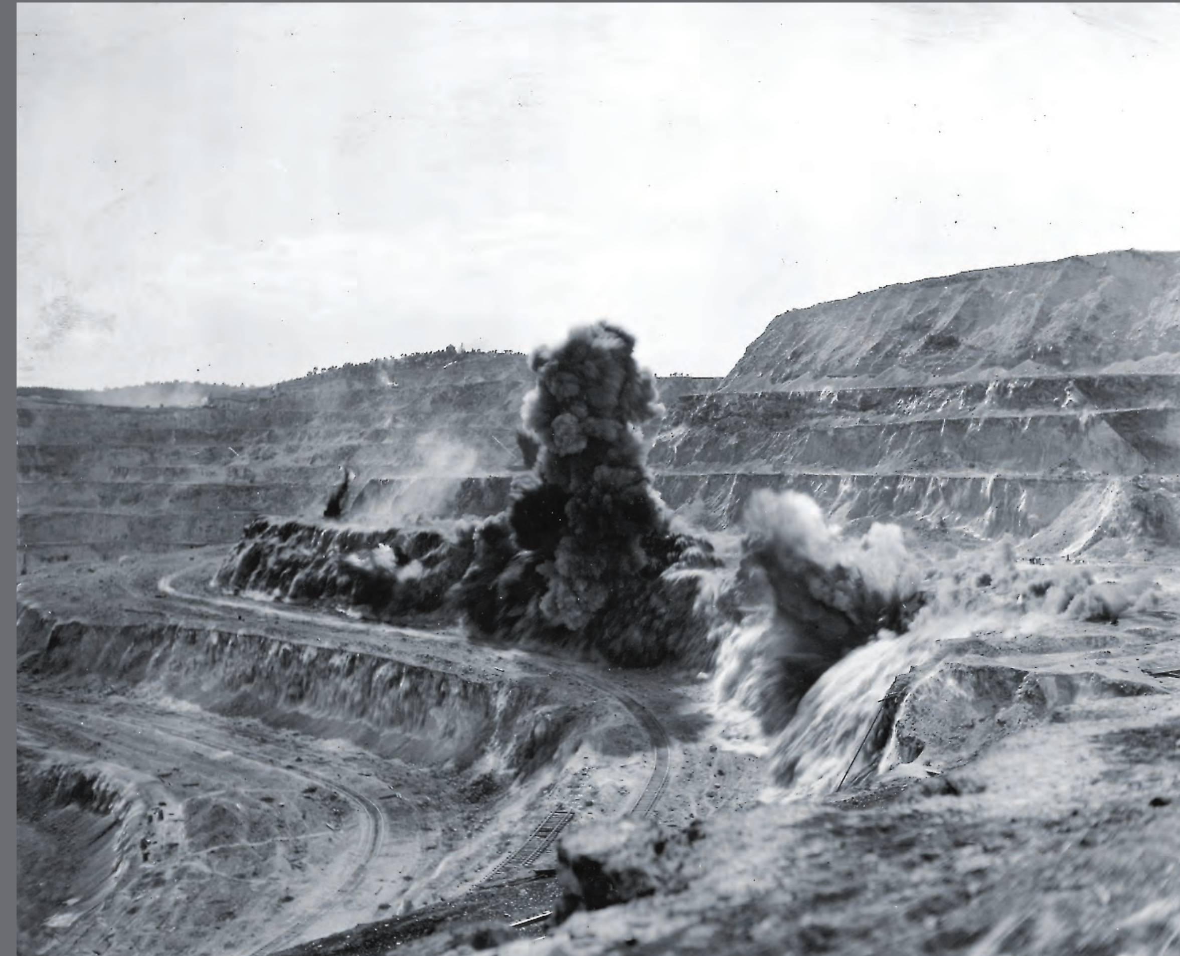
BLASTING ORE AND WASTE ROCK Miners expanded the Liberty Pit by blasting tall stepped “benches” down through the low-grade copper ore deposit as shown in this 1920s view. Huge amounts of waste rock containing little or no copper were hauled out of the pit to waste-rock dumps like Keystone Dump, which became a characteristic landform type of the open-pit mining process and landscape. Source: Nevada Historical Society
