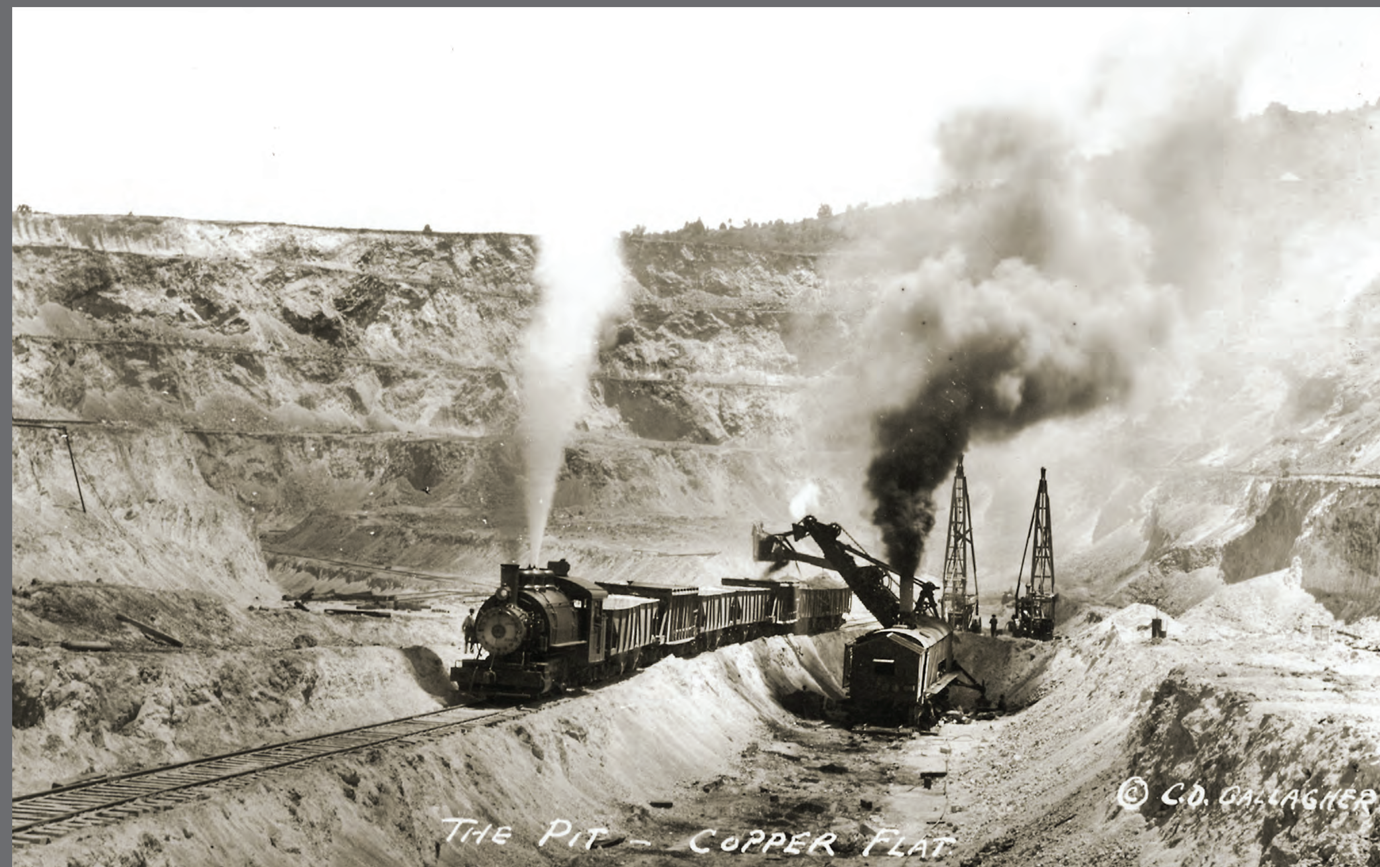
OPEN-PIT MINING MACHINES This World War I-era Liberty Pit image captures the working machines that made open-pit mining of porphyry copper ore deposits economical. The steam shovel in the trench at right is loading freshly blasted copper ore into a train of hopper cars that will take the ore to McGill for processing. At right, beyond the steam shovel, a pair of steam-powered “Keystone Drillers” are boring vertical holes for the placement of explosive charges to break up fresh ore for loading into the next train. Source: Nevada Historical Society
