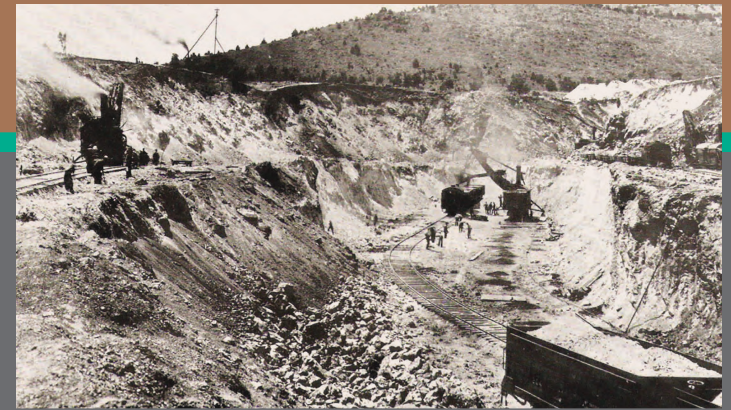
EARLY MINING AT THE LIBERTY PIT The Nevada Consolidated Copper Company began excavating the large, low-grade copper ore deposit at Ruth in 1907. NCCC used new "open-pit" mining methods with steam shovels and railroad trains to rapidly move large amounts of ore and waste rock. This operation, which became known as the Liberty Pit, was the third open-pit copper mine to open in the United States after Bingham Canyon, Utah, and Morenci, Arizona. Source: Memories of the Ruth Mining Area
