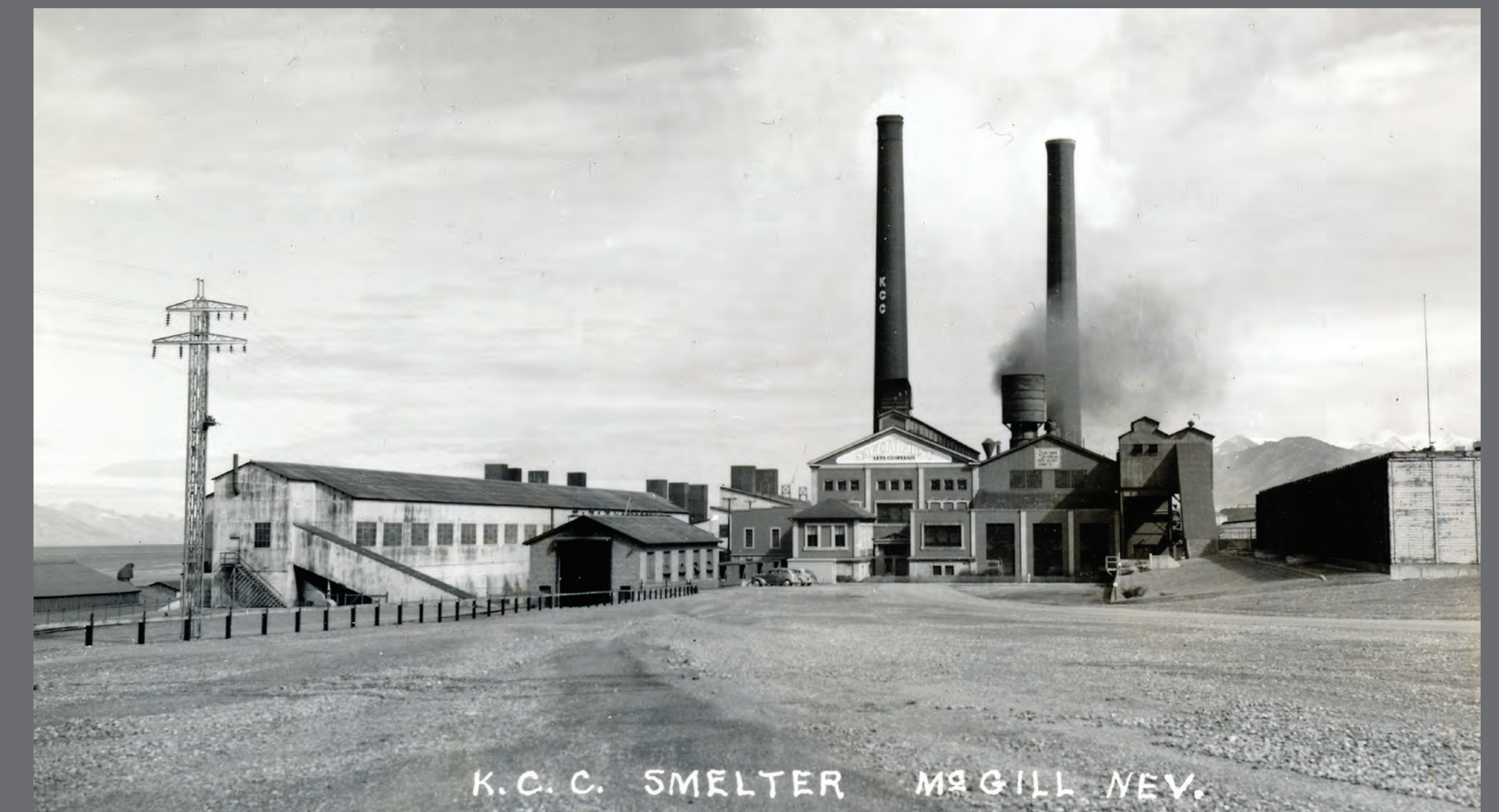
MCGILL REDUCTION WORKS At McGill, 20 miles northeast of Ruth, copper ore was concentrated and smelted to make impure "blister" copper that was refined in Baltimore, Maryland. This facility, shown here in the 1930s, was key to making Ruth copper mining profitable for Nevada Consolidated Copper and its successor, the Kennecott Copper Corporation. The works started producing copper in 1908 and closed in 1983. The surrounding town of McGill was one of two NCCC/KCC-owned "company towns" in the Robinson District. Source: Special Collections Department, University of Nevada, Reno Libraries
