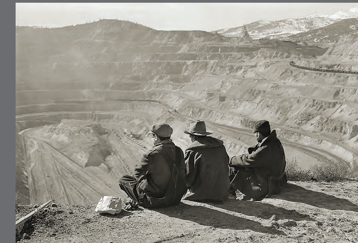
DUMPING WASTE ROCK AT KEYSTONE DUMP At first, mine dumps were built using trains of “dump cars” pulled by steam locomotives on movable tracks at the edges of the dumps. In 1948, Kennecott Copper introduced more-efficient diesel locomotives, and steam engines were taken out of service in 1950. In this image from the early 1950s, a diesel locomotive is on waste-rock duty on Keystone Dump, with three side-dump cars in action. In 1958, KCC ended railroad operations in the Liberty Pit and switched to more-efficient diesel trucks. Source: Nevada Historical Society
