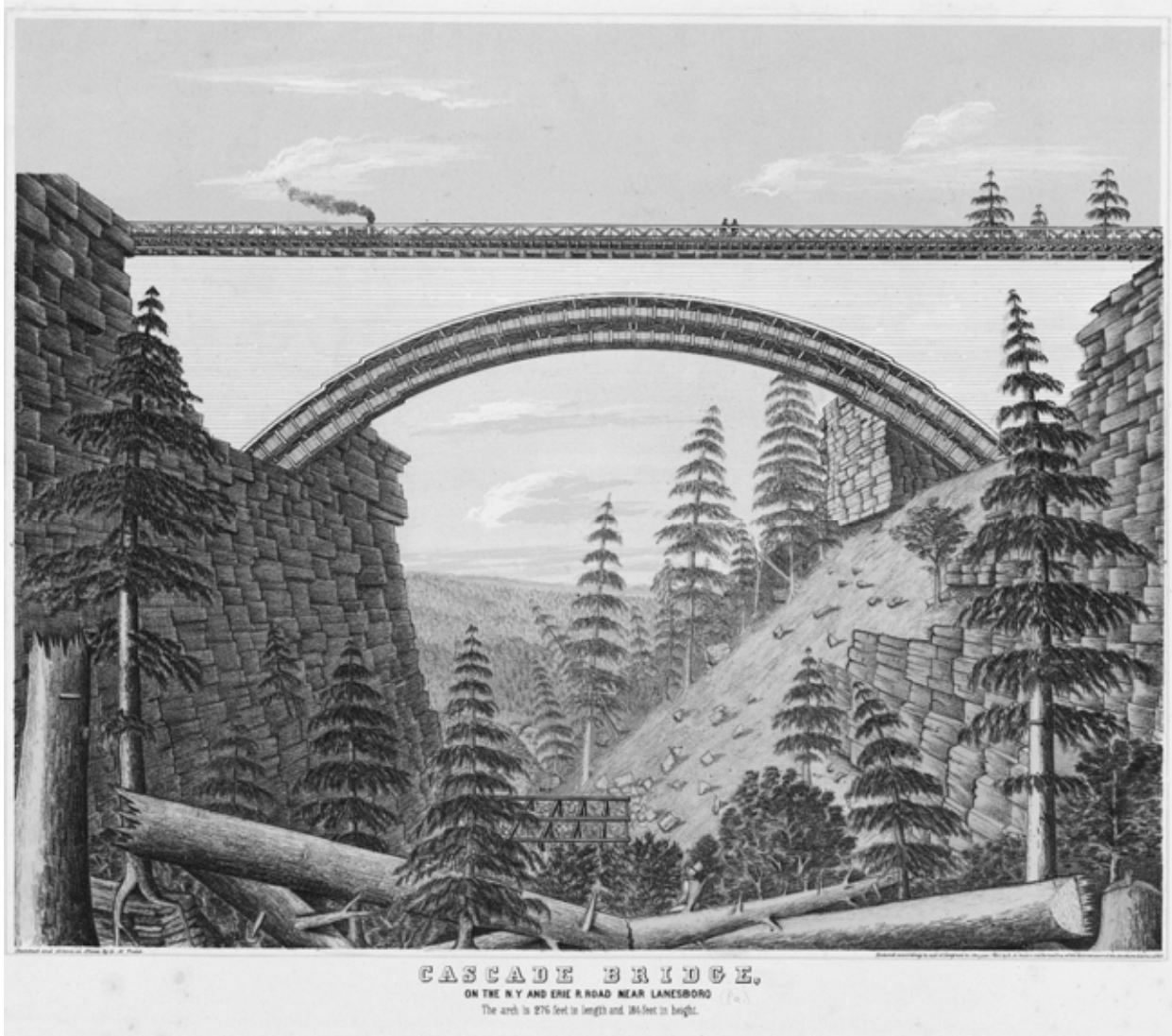
Figure 29. The Cascade Bridge, a 250' timber arch over Cascade Creek Gorge, near Lanesboro, Pennsylvania. Supported by eight 2'-wide white oak arch ribs, the bridge served the Erie from 1843-1860 when it was replaced by a massive fill. Library of Congress.
