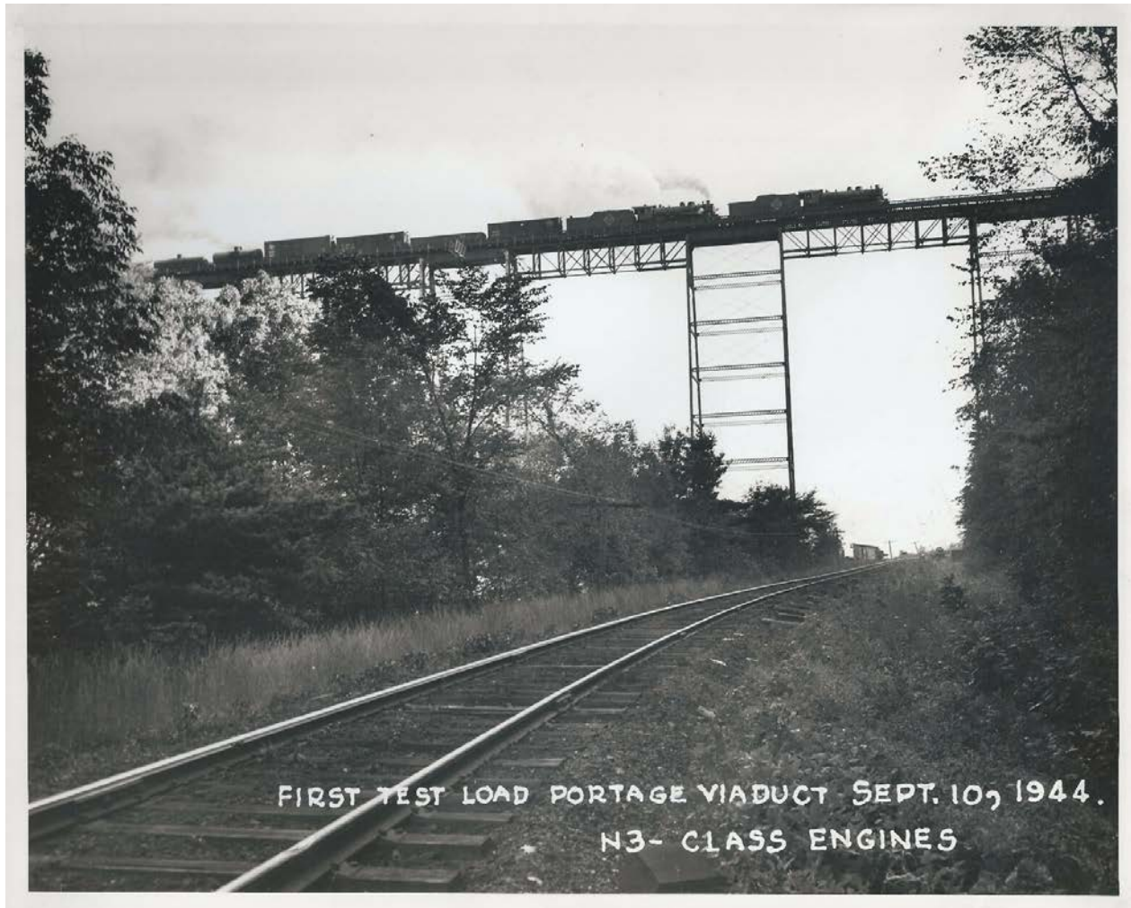
Figure 28. Double-headed Erie Railroad 2-8-2 Mikado steam locomotives lead the first test train across Portage Viaduct after the tower reconditioning project, September 10, 1944. The Pennsylvania Railroad's Rochester Branch runs under the bridge on the former Genesee Valley Canal alignment. Erie Railroad Photograph, E. S. Evans, Jr. Railway Photo. Matt Kierstead collection.
