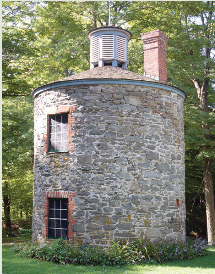
Wash and Change House where workers changed clothes before and after shifts, announced by a bell in the cupola. Source: Milestone Heritage Consulting
