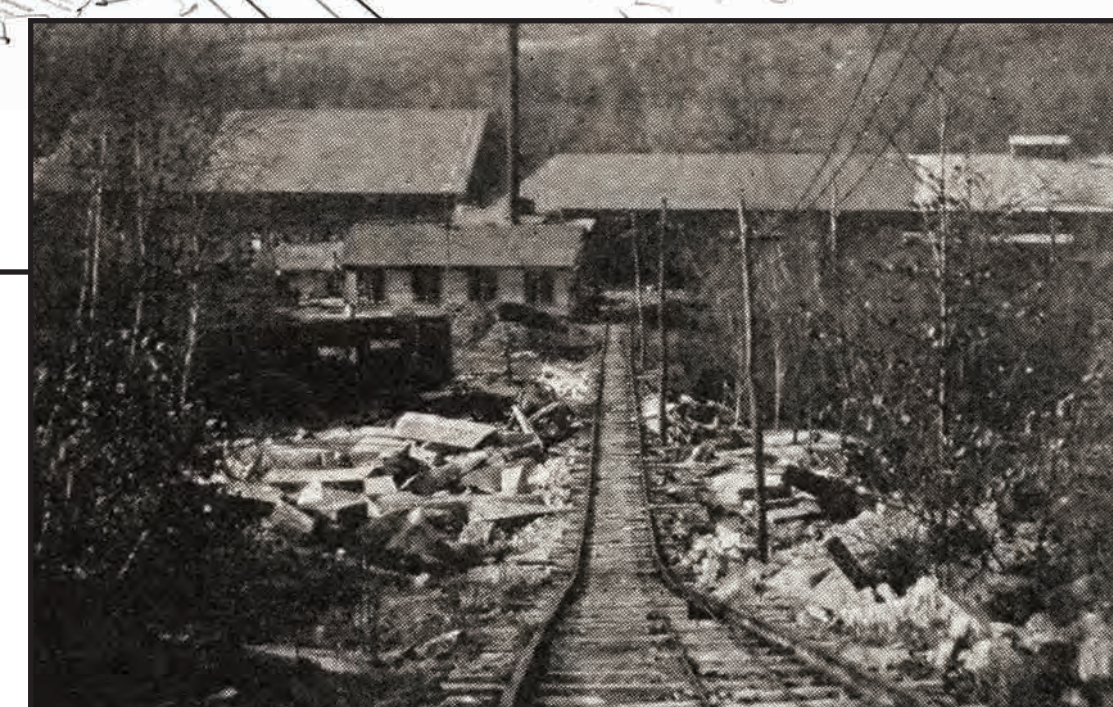
1920s MODERNIZATION | The quarry cutting and finishing sheds after the 1925-1927 Grenci & Ellis modernization. As part of the modernization, the incline railway tracks ran right into the new cutting shed housing the stone saws. Source: New York State Library.
