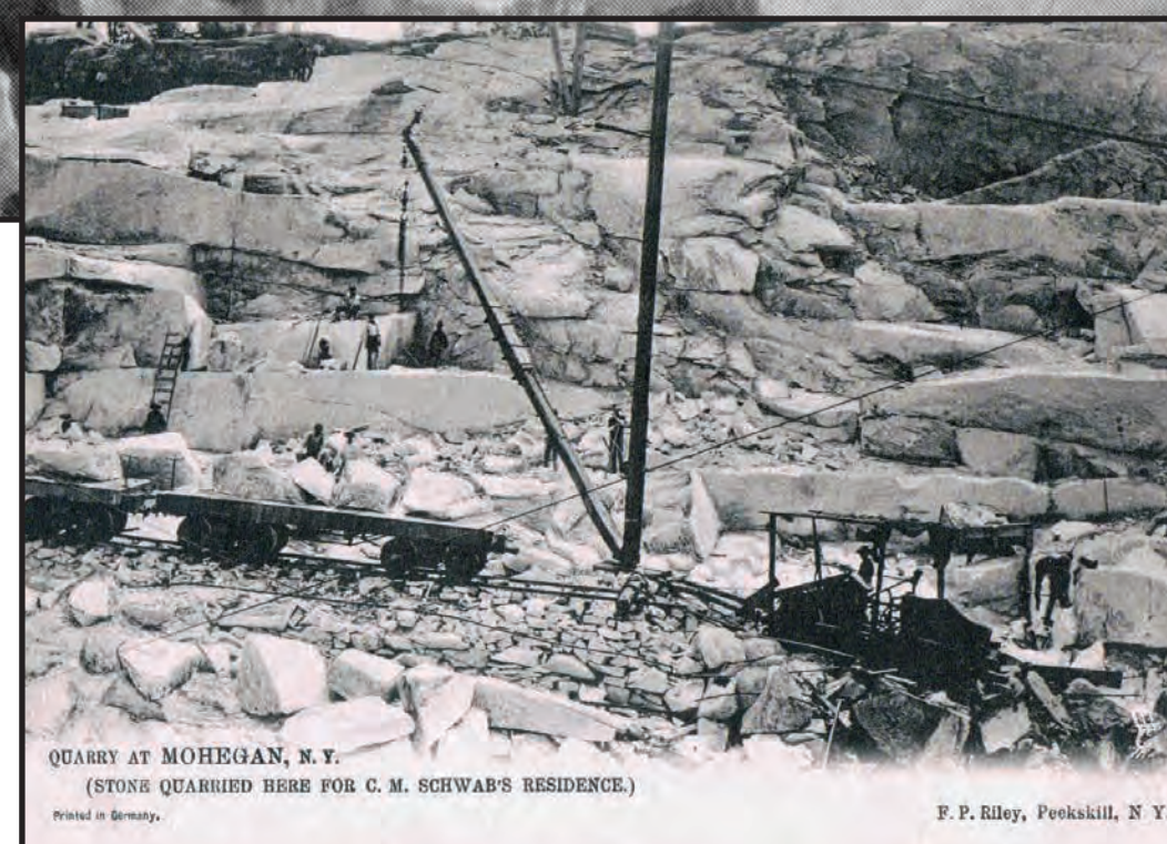
TEMPORARY DERRICK | This World War I-era postcard of the quarry shows a small, temporary derrick loading waste granite for disposal via a temporary railway. This photo clearly shows the natural horizontal and vertical splits in the rock that influenced how workers quarried it. Source: Dolores Pedi.
