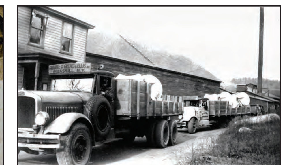
FINAL JOURNEY | Finished granite architectural ornaments leaving the Grenci & Ellis granite sheds on their fleet of delivery trucks in 1924. Source: Frank Goderre.
