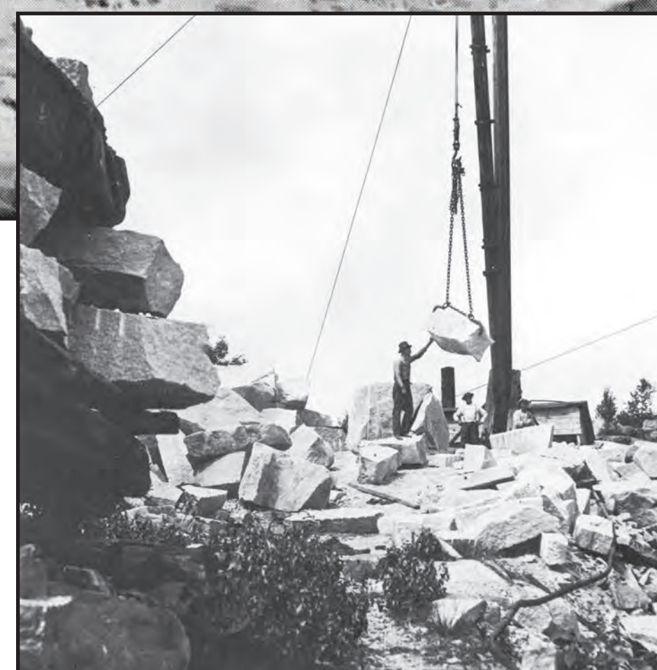
MOHEGAN QUARRY | A 1924 photograph of a large derrick at the edge of the quarry pit. Stones were lifted using chains and hooks called “lifting dogs” that gripped the notches chipped into each block, visible throughout the quarry today. A waste “grout” pile is visible at left. Source: Frank Goderre.
