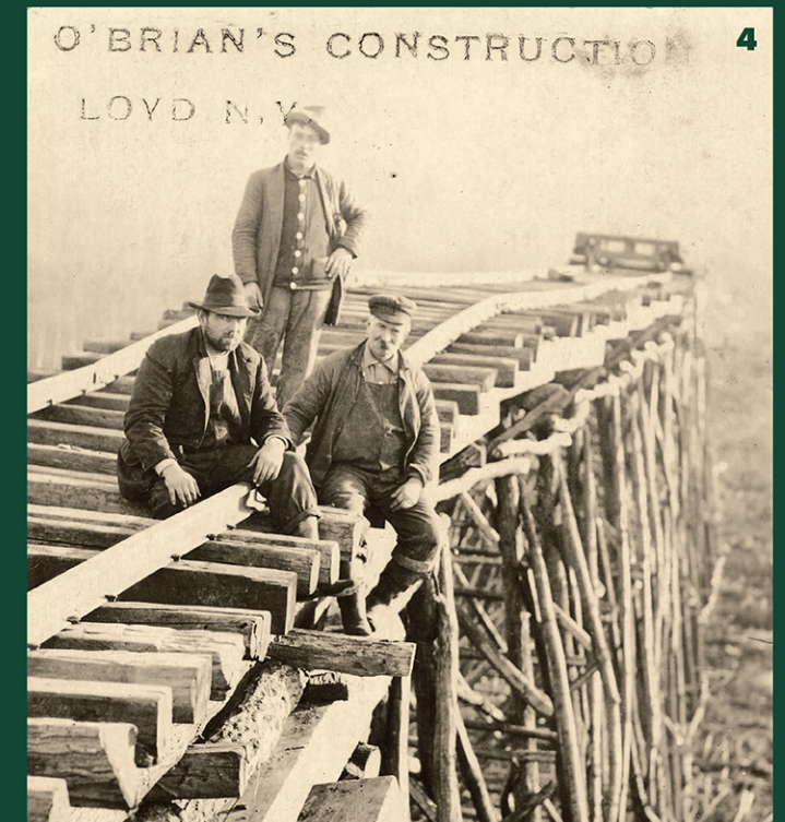
▲ RELOCATION CONSTRUCTION Postcards show 1912–1914 O'Brian's Construction Company Maybrook Line relocation work: 1. Steam drills at left made bedrock holes for placing explosives; smoke billows from a blast at right. 2. Steam shovels like this one at Centerville excavated railbed cuts through rock and soil. 3. Temporary timber trestle was used for dumping rock and soil from the cuts to build the embankment you are standing on; the 1889 track is visible at left. 4. Construction workers pose on the temporary trestle. Sources: John “Jack” Auchmoody and Vivian Yess Wadlin.
