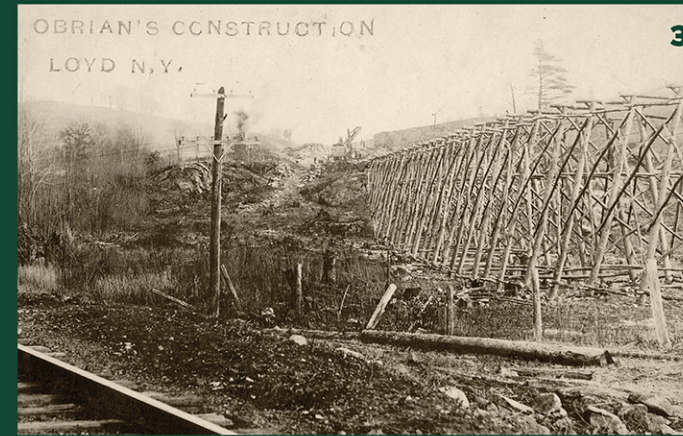
▲ RELOCATION CONSTRUCTION Postcards show 1912–1914 O'Brian's Construction Company Maybrook Line relocation work: 1. Steam drills at left made bedrock holes for placing explosives; smoke billows from a blast at right. 2. Steam shovels like this one at Centerville excavated railbed cuts through rock and soil. 3. Temporary timber trestle was used for dumping rock and soil from the cuts to build the embankment you are standing on; the 1889 track is visible at left. 4. Construction workers pose on the temporary trestle. Sources: John “Jack” Auchmoody and Vivian Yess Wadlin.
