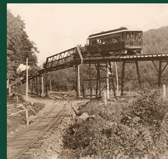
▲ TROLLEY BRIDGE The 1897–1925 New Paltz–Highland electric trolley line followed New Paltz Road and passed over the Maybrook Line on this steel viaduct at Brooks Crossing until the railroad and overpass were relocated northeast in 1914. Illinois Mountain rises in the background. Source: Town of Lloyd Historian's Collection.
