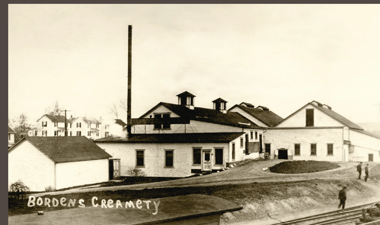
▲ BORDEN'S CREAMERY Built southwest of the depot by the New York Condensed Milk Company in 1901, this rail-served Hopewell Junction plant processed three thousand gallons of local dairy milk per day, shipping it to distributors in insulated boxcars kept cold with winter ice cut from local ponds. Source: David Turner.
