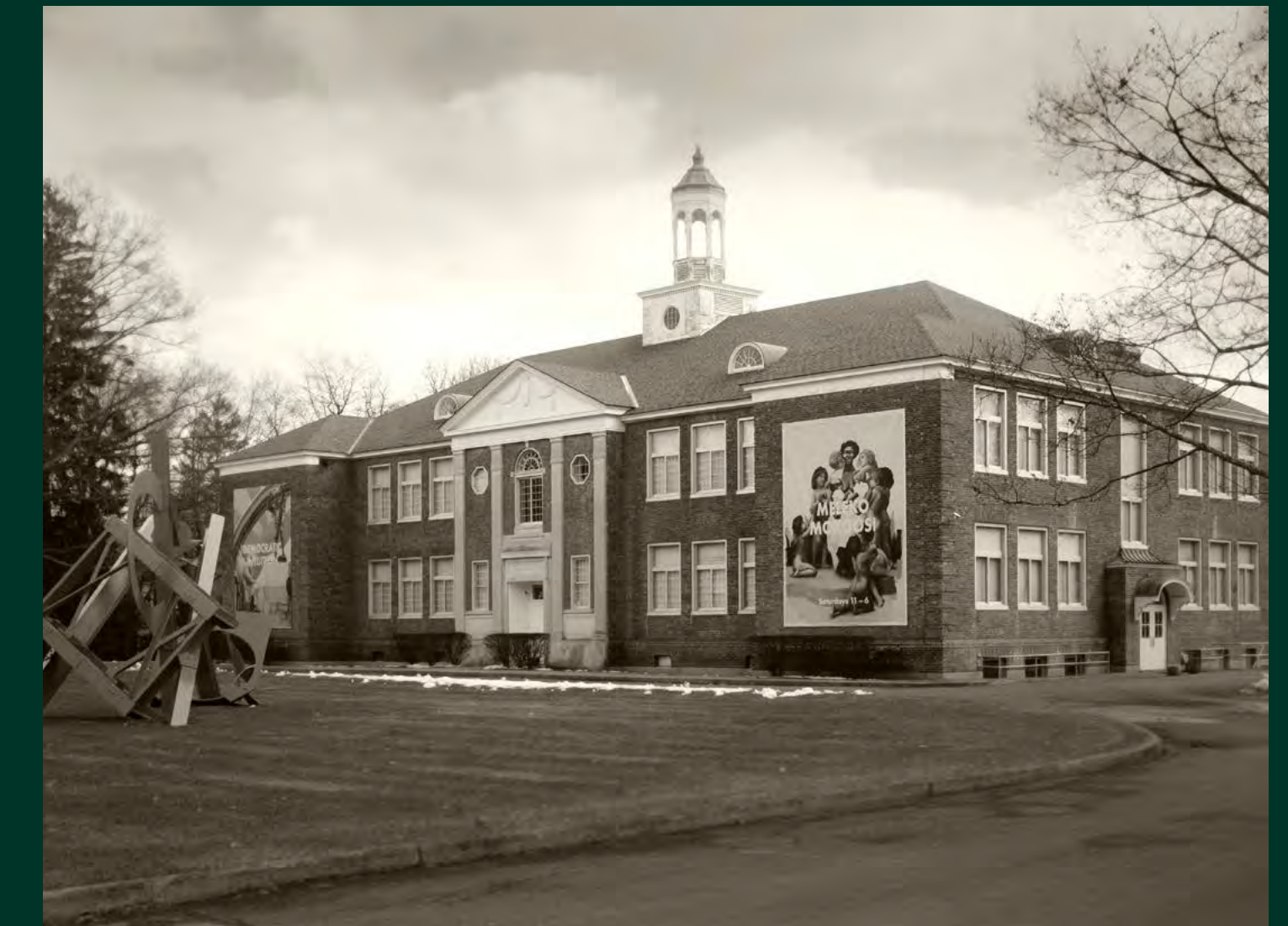
MARTIN VAN BUREN SCHOOL , 25 Broad Street (1930) This Colonial Revival-style school was dedicated by Franklin Delano Roosevelt. Built for kindergarten to Grade 12 students, it is now a contemporary art gallery. Source: Milestone Heritage Consulting.
