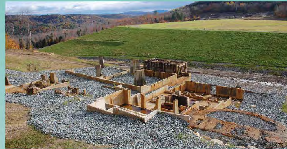
Cleared and preserved World War II copper ore mill foundations, with completed mine waste storage area visible beyond. Source: U.S. Environmental Protection Agency.
