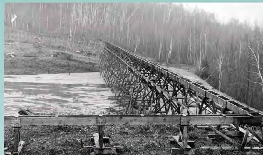
Left: A miner poses with an electric mine locomotive, 1950s. Source: Strafford Historical Society. Below: Elevated wood troughs for pumping copper mill waste onto the tailings pile, 1950s. Source: Strafford Historical Society.
