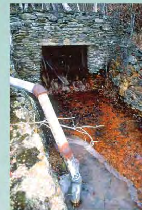
Contaminated water flowing from the Elizabeth Mine 1898 adit (entrance tunnel), 2003. Source: U.S. Environmental Protection Agency.
