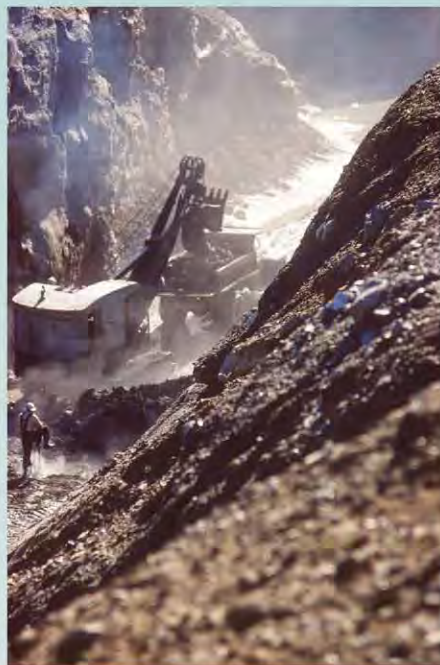
Excavating copper ore from the South Open Cut, early 1950s. Source: Strafford Historical Society.
