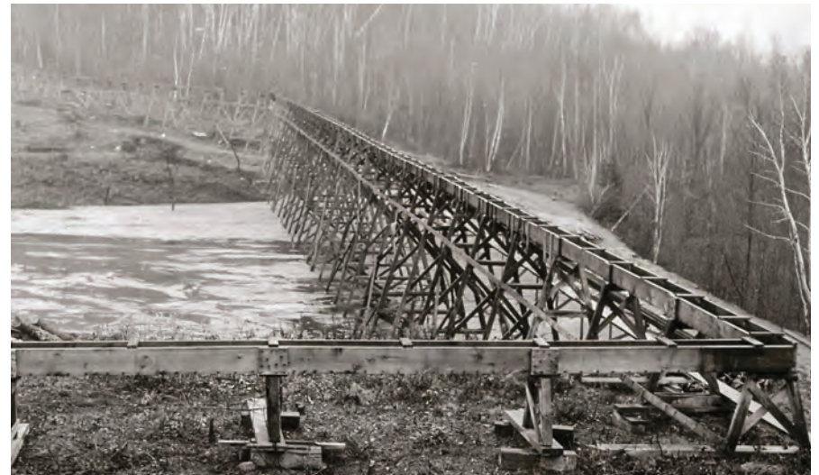
The unwanted ground waste tailings were pumped away from the flotation mill in a liquid slurry through a “launder”—a series of pipes and troughs that led out to the tailings pile. Source: Strafford Historical Society.
