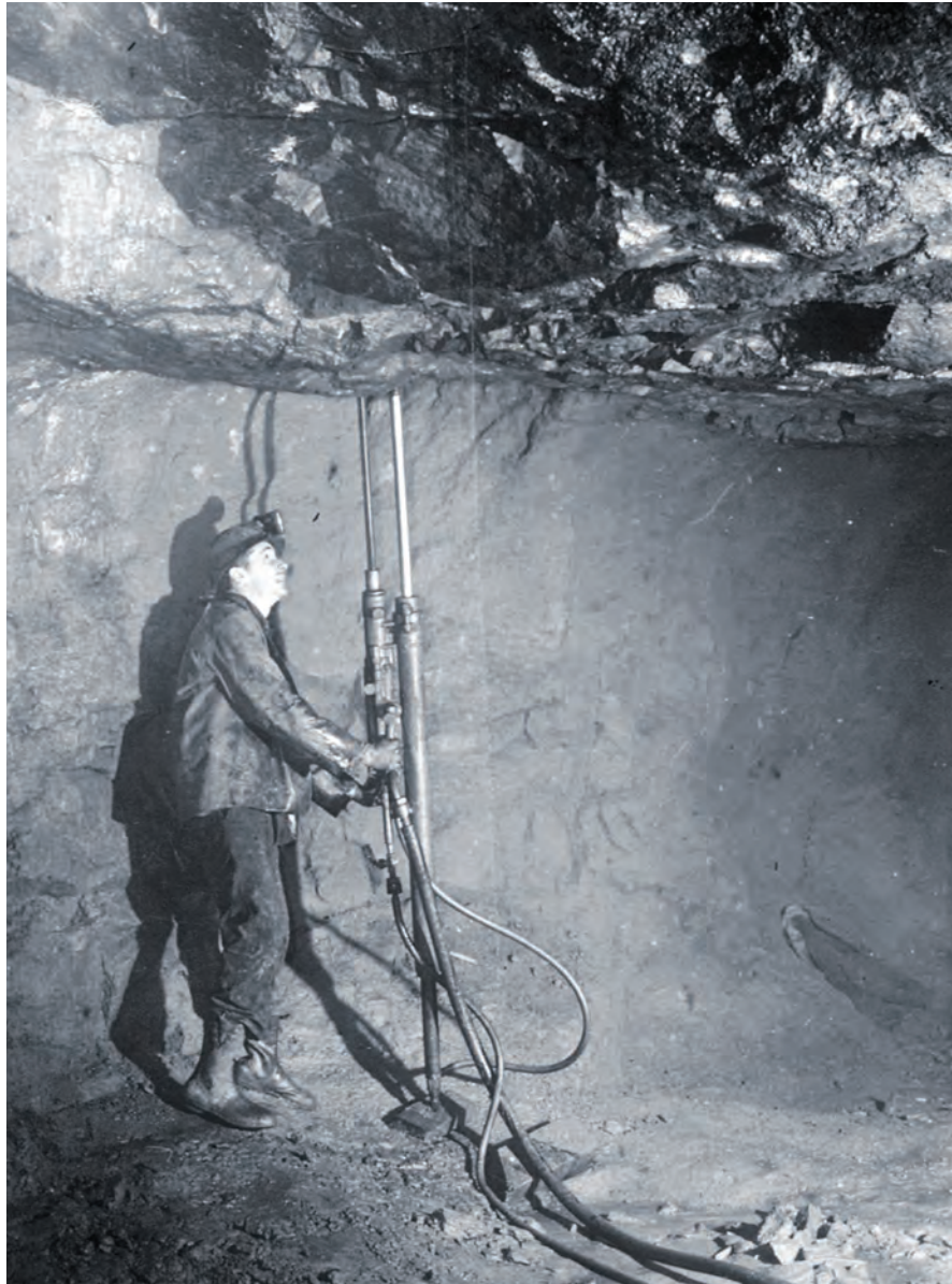
Elizabeth Mine, 1950s scene of miner drilling overhead with compressed-air drill. Source: Strafford Historical Society.
