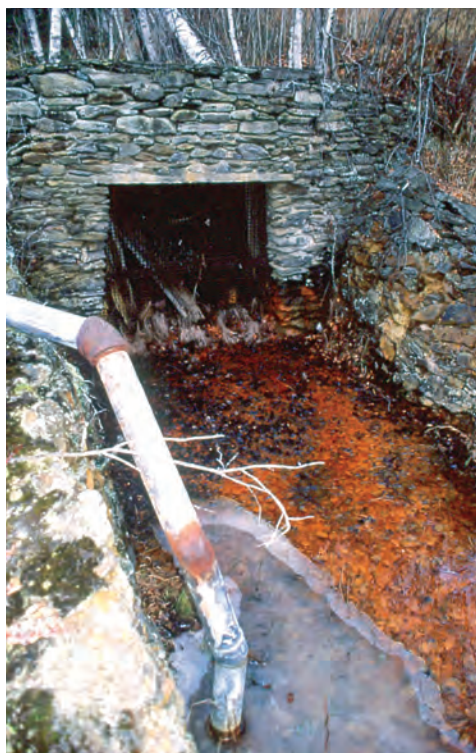
Acid mine drainage flowing from the 1898 Tyson adit, 2003. Source: U.S. Environmental Protection Agency.
