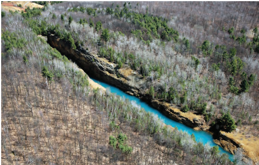
South Open Cut looking northeast in 2007, with portion of copperas works area at upper left. The 1,600-foot-long cut was surface mined for copper ore from 1950 to 1953. Runoff from the cut and nearby South Mine contributed copper to the watershed of Lord Brook, also a tributary of the Ompompanoosuc, and ultimately, the Connecticut River. Source: U.S. Environmental Protection Agency.
