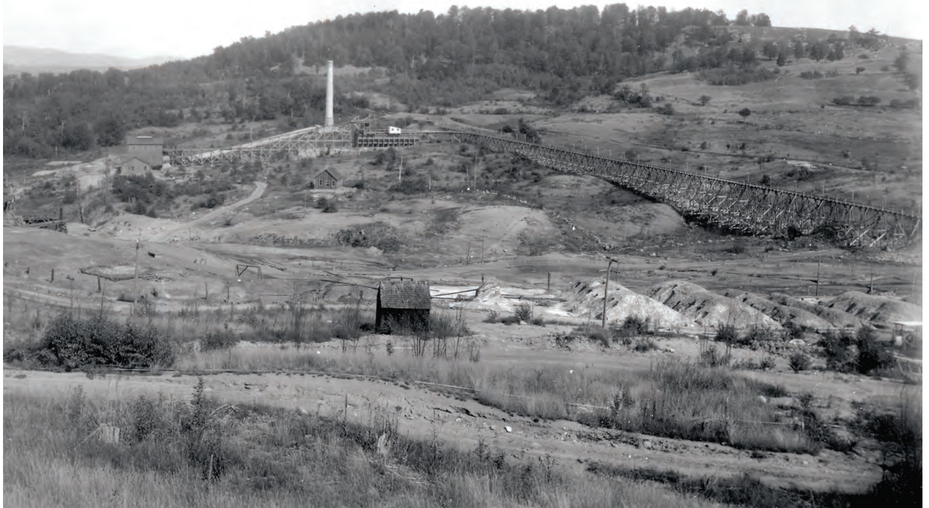
August Heckscher's Vermont Copper Corporation smelting plant about 1908. Ore was transported over the trestle at right and across to the smelter at left. Flue and chimney were for dispersing smelter fumes. Ore roast beds from the Tyson family's previous Elizabeth Mining Company smelting operation are in foreground. Source: Strafford Historical Society.
