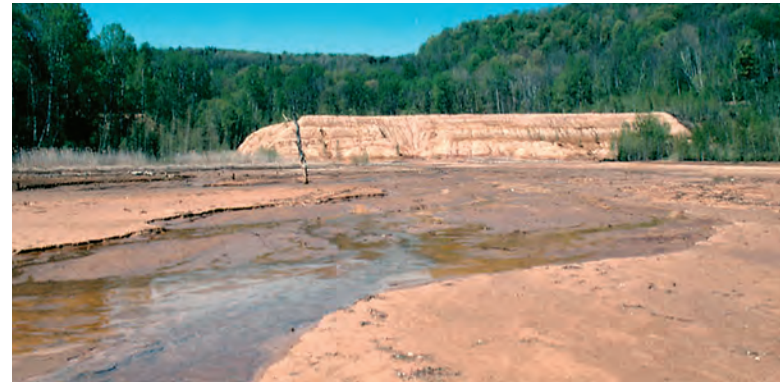
View from 2003 looking southwest across larger tailings pile to smaller one deposited when pyrrhotite extraction began in 1951. Water flowing through the tailings discharged dilute sulfuric acid and up to 800 pounds of dissolved iron a day into Copperas Brook. Source: U.S. Environmental Protection Agency.
