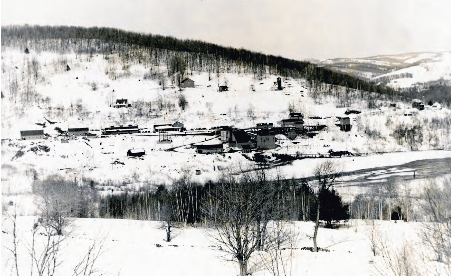
Panoramic 1940s winter view of the Vermont Copper Company's World War II Elizabeth Mine plant looking west, showing, from left to right: miners' change house, air compressor building, machine shop, office/warehouse, and the mill complex including garage, ore storage bin, flotation mill, thickener/dryer building, and crusher. The water tank building and 1948 shaft hoist house and head frame are on the hill at center, and the infirmary and clubhouse at the extreme right. The gently sloping mill tailings pile fills the valley in the foreground. For additional information see documentation drawings on pages 54 through 57. Source: Strafford Historical Society.
