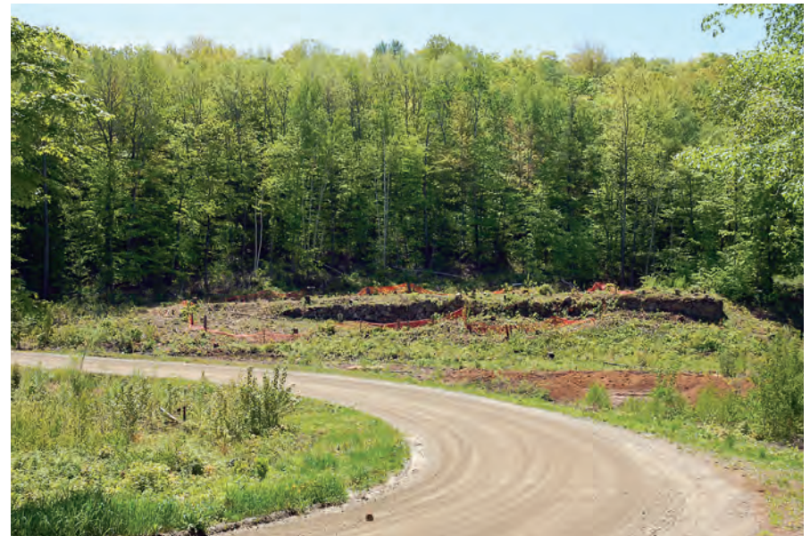
Lower copperas factory foundation on Mine Road, 2009. Copperas manufacturing from 1809 to 1882 involved lead-lined vats and plumbing, which left small but highly lead-contaminated areas in and immediately around the two factory foundations. Source: U.S. Environmental Protection Agency.
