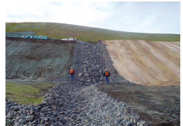
The top and sides of the sealed cap were covered with over two feet of soil, which was treated with lime, fertilized, and planted with grass. Rock-lined trenches divert surface runoff off and around the cap. Water filtration has been reduced so that the tailings now discharge less than 100 pounds of dissolved iron per day — about 88 percent less than the peak discharge of 800 pounds per day. Source: U.S. Environmental Protection Agency.
