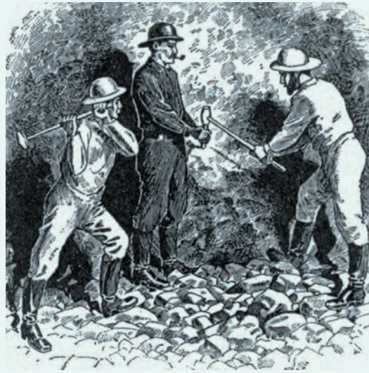
Miners using a manual drill and sledgehammers to bore a hole in rock. Source: International Correspondence Schools, 1907.
