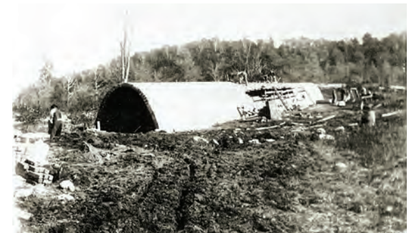
Vermont Copper Corporation brick-arch smelter smoke flue under construction, about 1908. Source: Strafford Historical Society.
