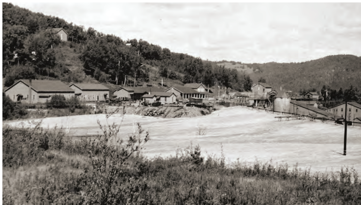
Mine plant looking northwest in the 1950s. The foreground tailings pile was the second one created, south of the first, after separation of the pyrrhotite in the ore for the Brown Paper Company began in 1951. Source: Strafford Historical Society.
