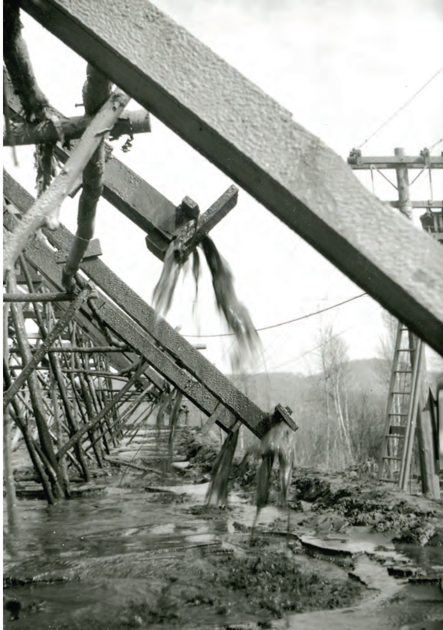
A 1948 photograph shows ore mill tailings flowing out of the movable launder at the front edge of the ever-expanding tailings pile, which eventually filled the Copperas Brook valley and became the largest landscape feature associated with the 1943–1958 operations. Source: Strafford Historical Society.
