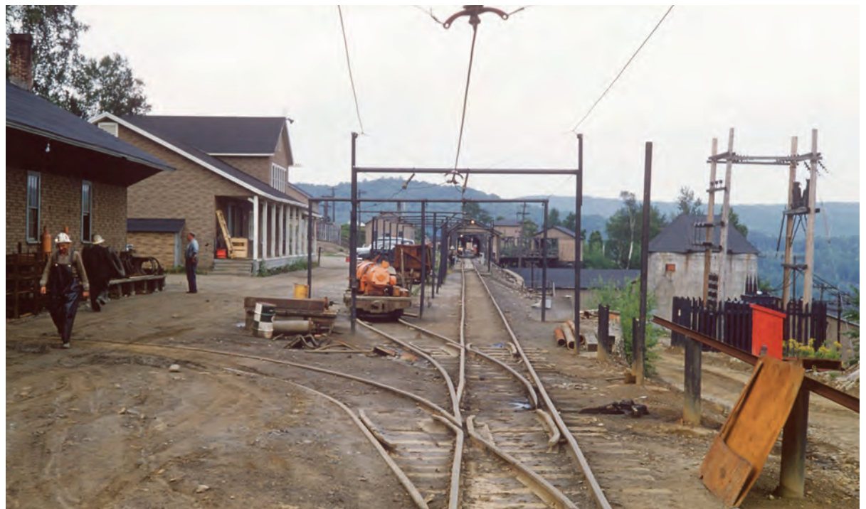
View looking north along the mine surface railroad, in the 1950s. Spur track at left leads into the machine shop, where mine locomotives, ore cars, and heavy equipment were serviced and repaired. The round concrete ore storage bin for the processing mill is at right. Source: Strafford Historical Society.
