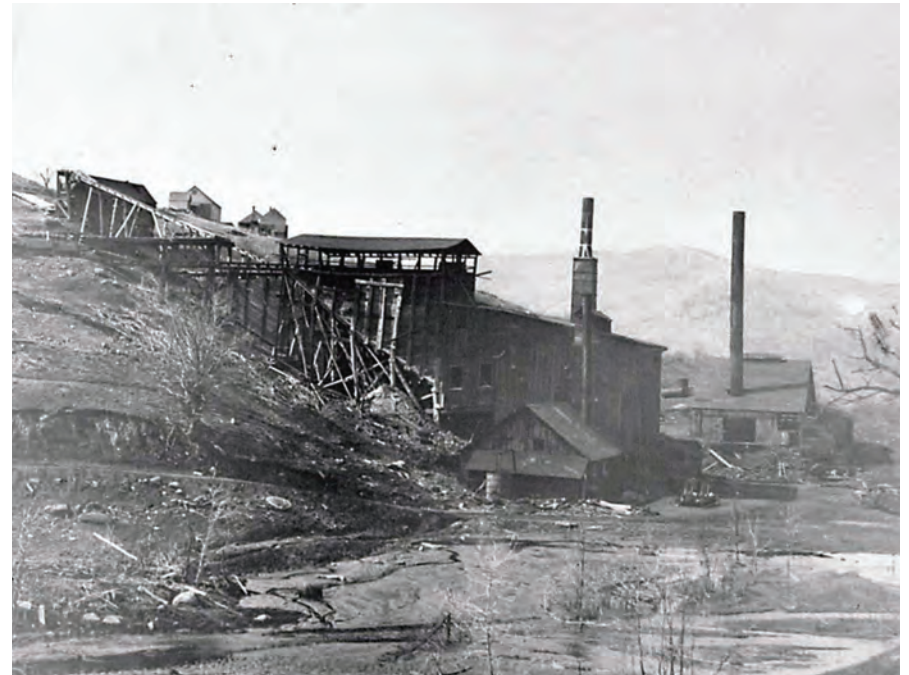
Tyson mill and roast beds, about 1900. The mine railroad trestle was used for delivering ore to roast beds. Sulfur fumes can be seen rising from roasting ore. Source: Collamer Abbott Collection, University of Vermont.
