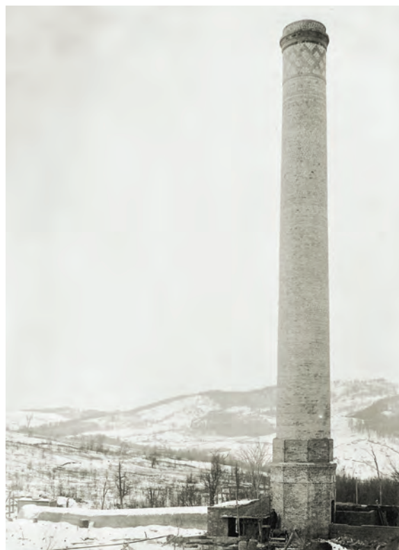
Vermont Copper Corporation smelter chimney under construction, about 1908. The chimney was intended to disperse smelter fumes in the valley. Source: Strafford Historical Society.
