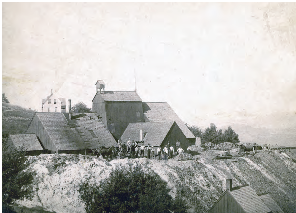
Miners pose outside the cluster of buildings above the No. 1 shaft on Copperas Hill, 1880s. These buildings housed the steam engine, hoist, and ore crusher. Source: Collamer Abbott Collection, University of Vermont.
