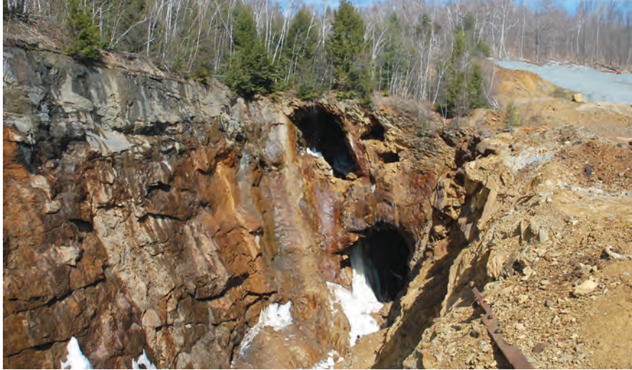
North end of 1,000-foot-long North Open Cut looking north, showing open stopes (chambers) where mining extended north underground, 2010. Source: U.S. Environmental Protection Agency.
