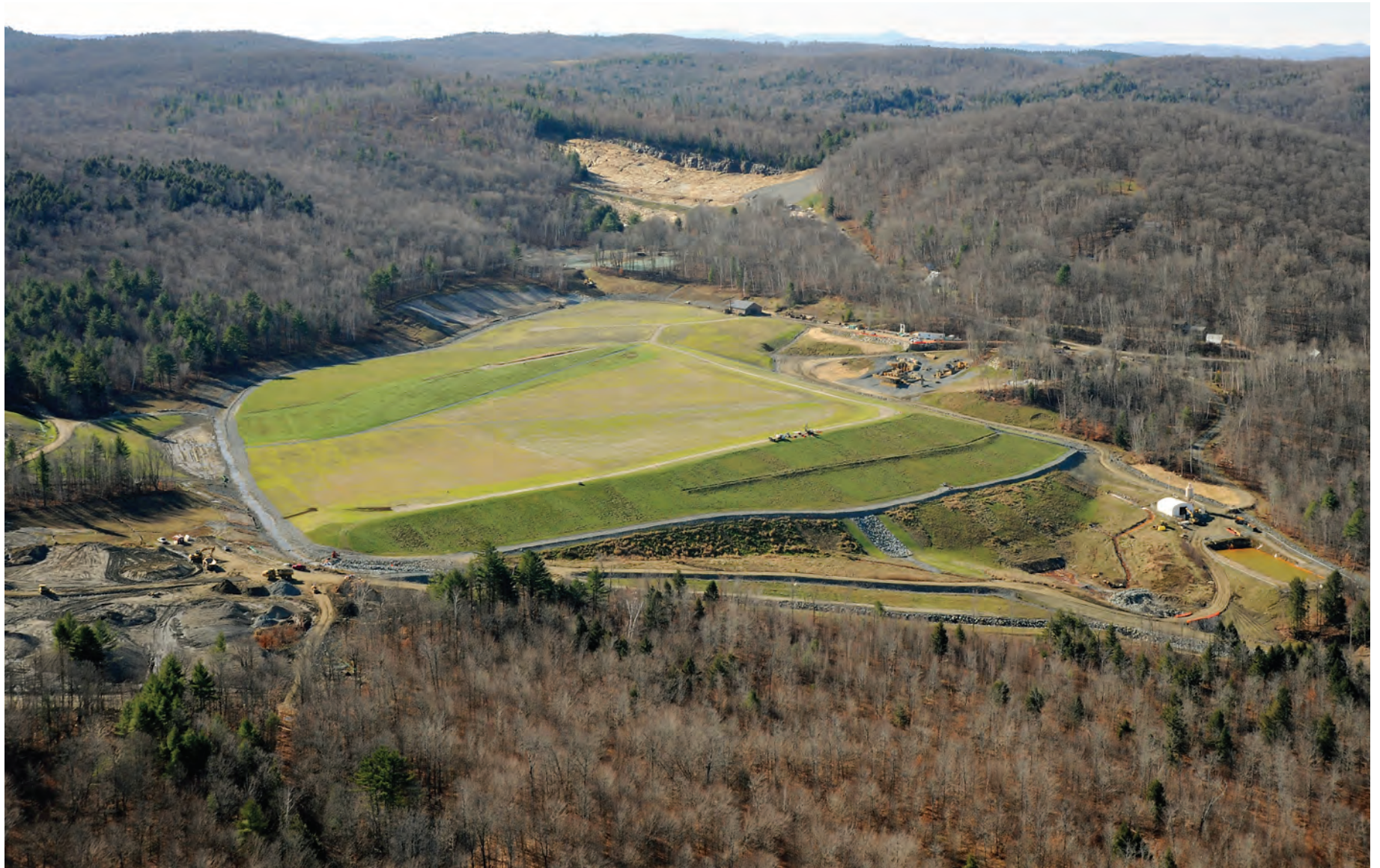
Elizabeth Mine looking southwest, 2012. The 1943–1958 ore mill tailings, named tailings piles (TP) 1 and 2 by the EPA, became the repository platform for over 356 thousand cubic yards of consolidated mine waste, excavated from Mine Road, the South Mine, the South Open Cut, the copperas factories, the TP-1 and TP-2 perimeter, and the copperas works roast beds / heap leach piles (TP-3), visible in the background below the North Open Cut. Source: U.S. Environmental Protection Agency.
