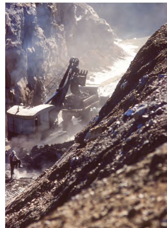
Cable shovel excavating copper ore from the South Open Cut in the early 1950s. Source: Strafford Historical Society.
