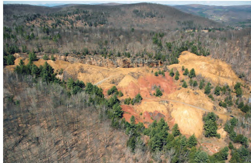
Copperas Hill looking west in 2009 showing North Open Cut at center. The 1880s–1890s Tyson mining area is at center right, reddish copperas manufacturing roast beds / heap leach piles with Copperas Road are at center, and upper copperas factory site is at lower right. Source: U.S. Environmental Protection Agency.
