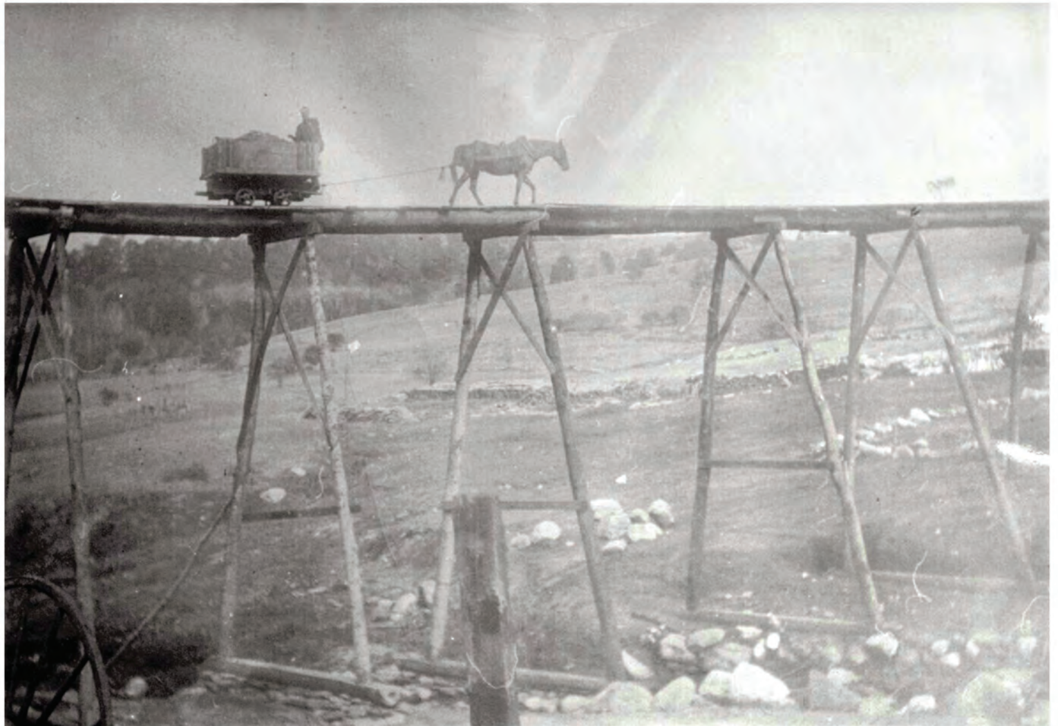
Elizabeth Mine, horse hauling ore car and miner on trestle, 1890s. Source: Strafford Historical Society.
