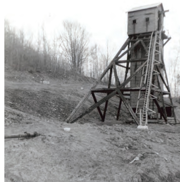
Headframe tower for the 1948 shaft. Cables from the hoist room ran over grooved sheave wheels, or pulleys, at the top of the tower and were attached to the ore skip and man cage that traveled up and down the shaft to the 975-foot level. Source: Strafford Historical Society.
